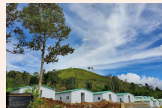
Temporary Camp of Dairi Project
