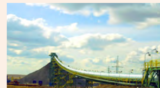
Bozshakol Project Corridor
