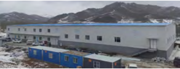
CNBM utilizes coal mine drainage for beneficiation production and uses high-pressure water from pipelines under coal mine to supply water equipment and facilities for tasks like underground rock drilling and dust reduction, with approximately 9,000 tons of water being saved per day.
