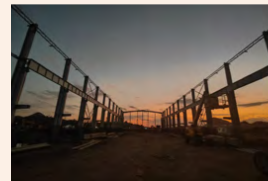
Steel Structure Installation for the Potroom of the Indonesia ACCS Project
