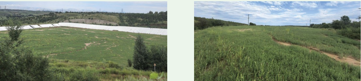
Hazardous Waste Storage Site Upon Completion of Pollution Prevention Project ^
